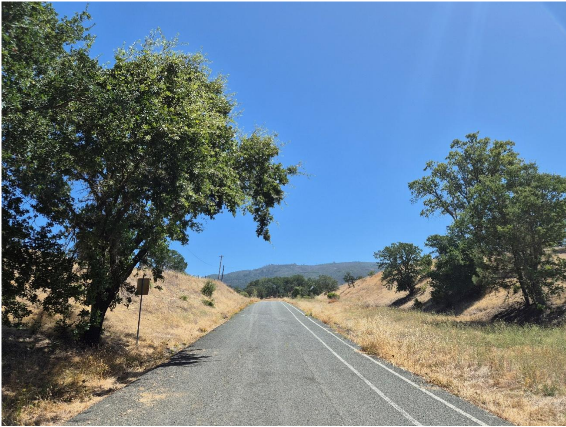
Caption: A photograph of Sunrise Road on the east side of the Sonoma Developmental Center Open Space property. Photograph by: Carmen Vanni, California State Parks
