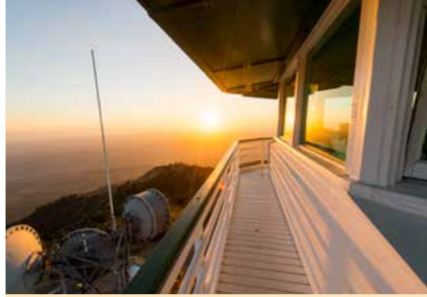
Boucher Hill Fire Lookout Tower
